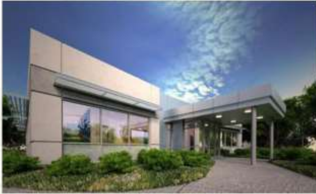
Joint Personal Support Unit, Halifax
