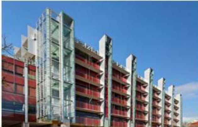
Computer Sciences Building , Adelaide
